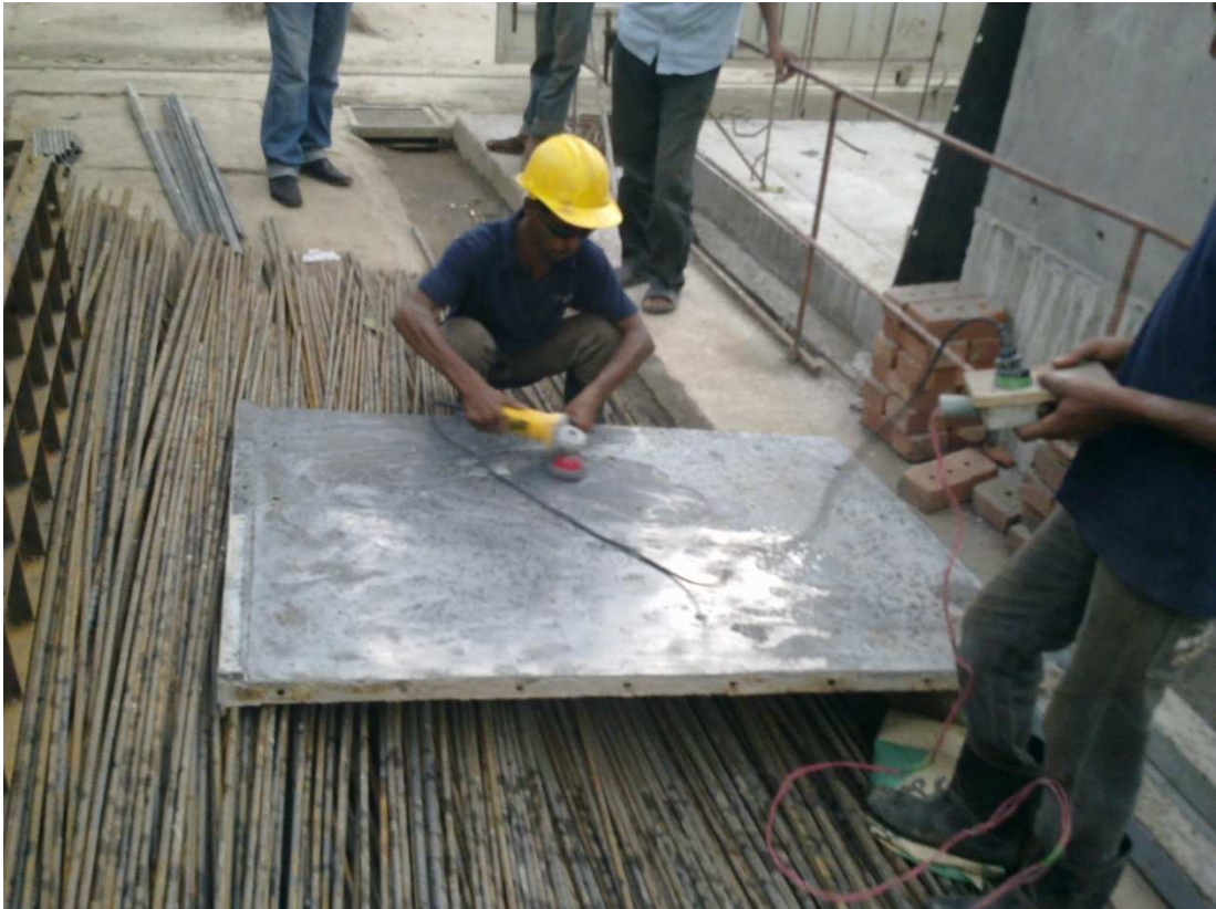
MS Shutter is cup brushing for better concrete surface
